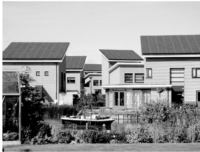
Figure 6.18: Houses in Langedijk with PV modules mounted on the roofs.
